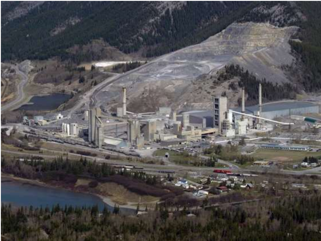
Canada's Lafarge cement plant at Exshaw near Canmore. Photo by Postmedia Archives
